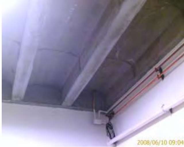
Typical Cast-in-Place Concrete Intermediate Floor
