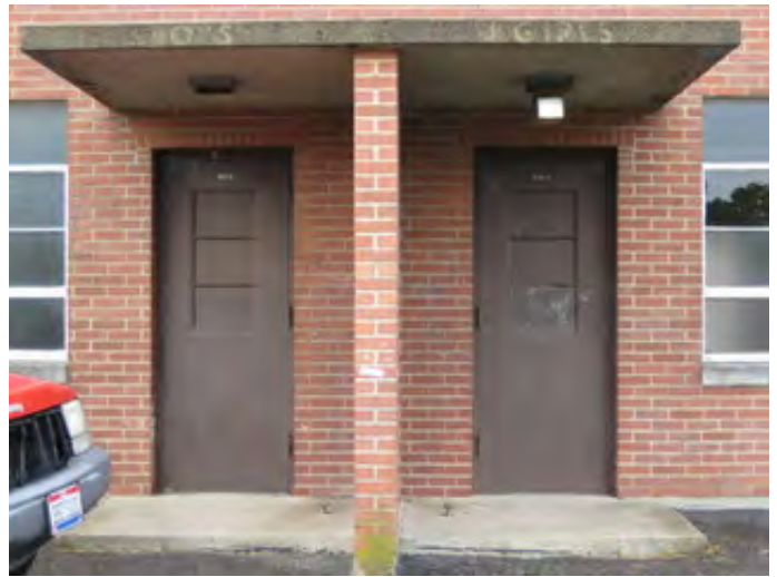
Typical Exterior Doors
