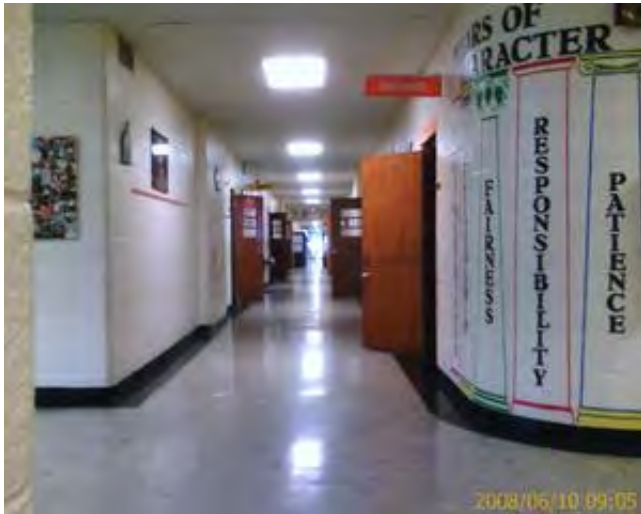
Typical Corridor Condition
