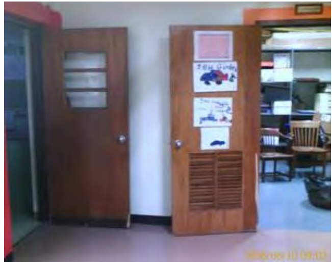
Typical Door Condition
