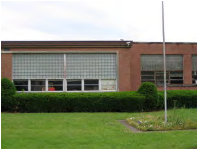
Typical Aluminum Frame Windows with Glass Block
