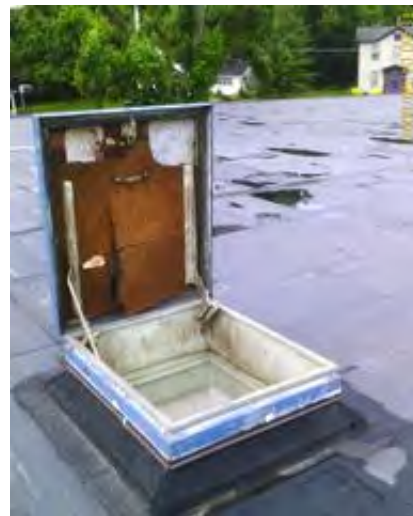
Typical Roof Hatch Condition
