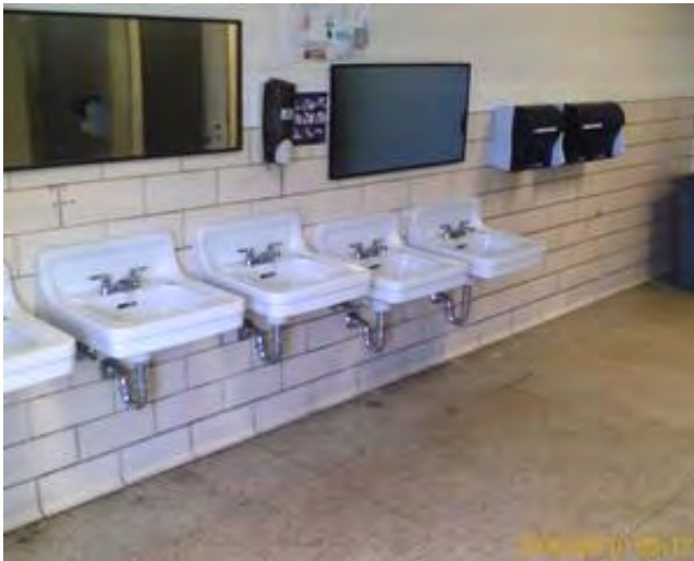
Typical Fixture Condition
