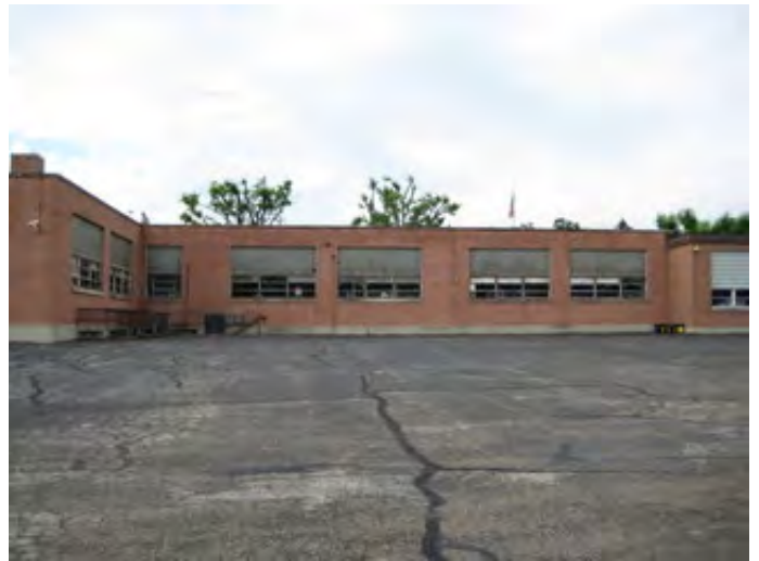
Typical Steel Frame Windows with Glass Block
