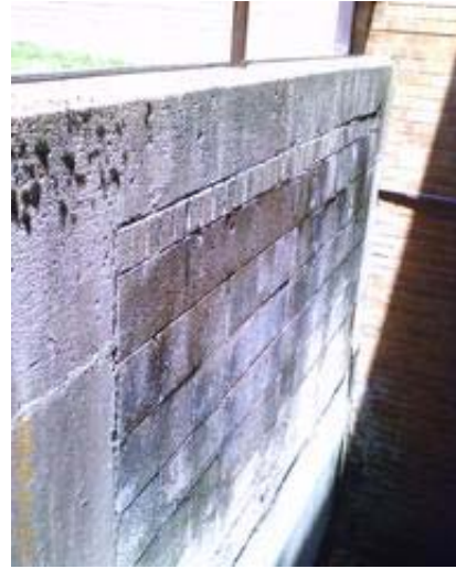
Typical Masonry Foundation Wall
