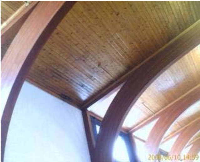
Typical Gymnasium Roof Structure
