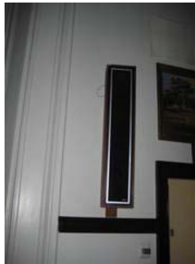
Specialized Stage Sound Equipment
