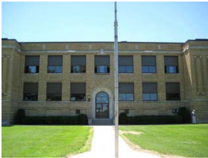
Typical Aluminum Frame Windows
