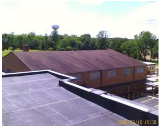
Typical Asphalt Shingle Roof
