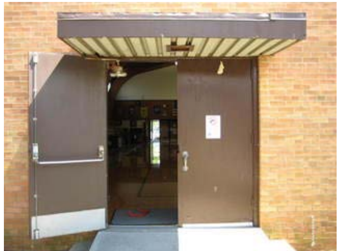
Typical Exterior Doors
