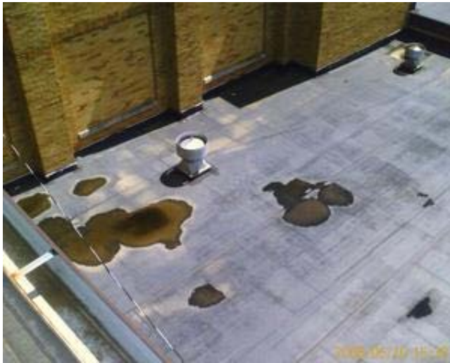
Typical EPDM Roofing Condition
