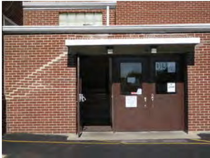
Typical Exterior Doors
