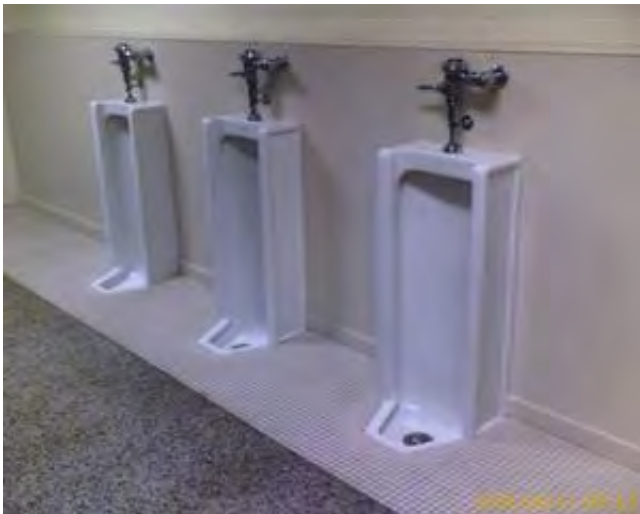
Typical Floor Mounted Urinals
