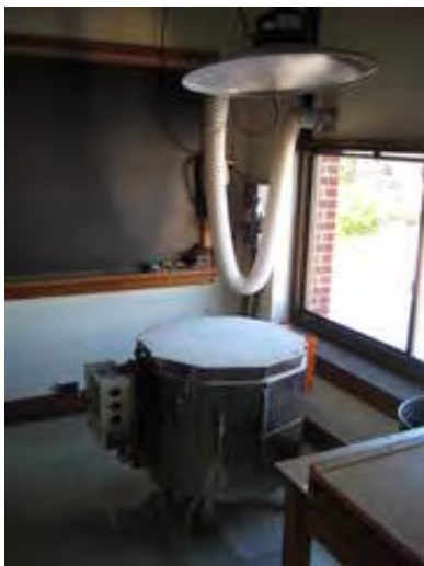
Art Program Kiln Exhaust System
