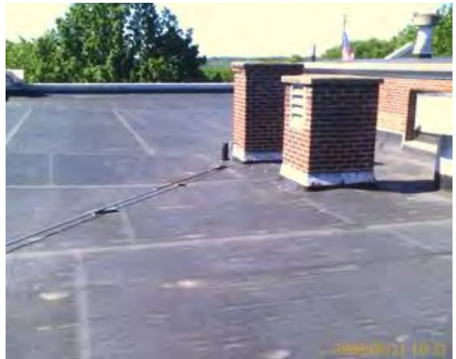
Typical EPDM Roofing Condition
