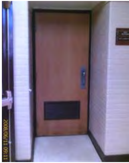
Typical Narrow Recessed Door
