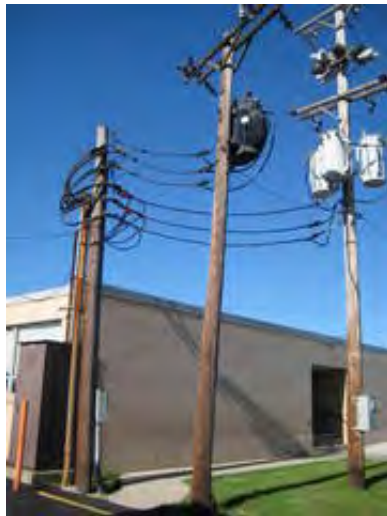
Pole-Mounted Transformers
