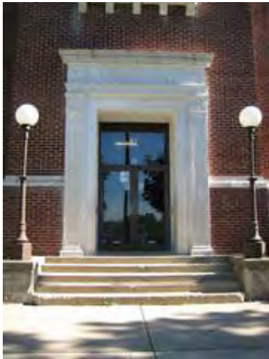
Main Entrance Doors
