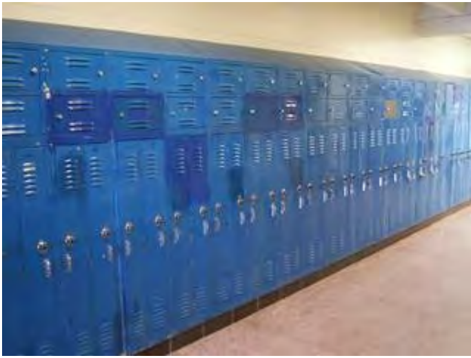
Typical Corridor with Lockers in Poor Condition
