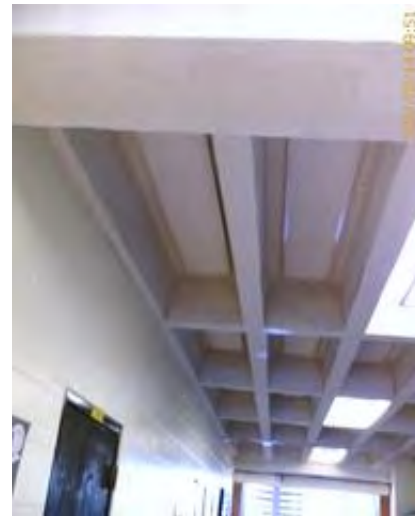
Typical Cast in Place Concrete Intermediate Floor
