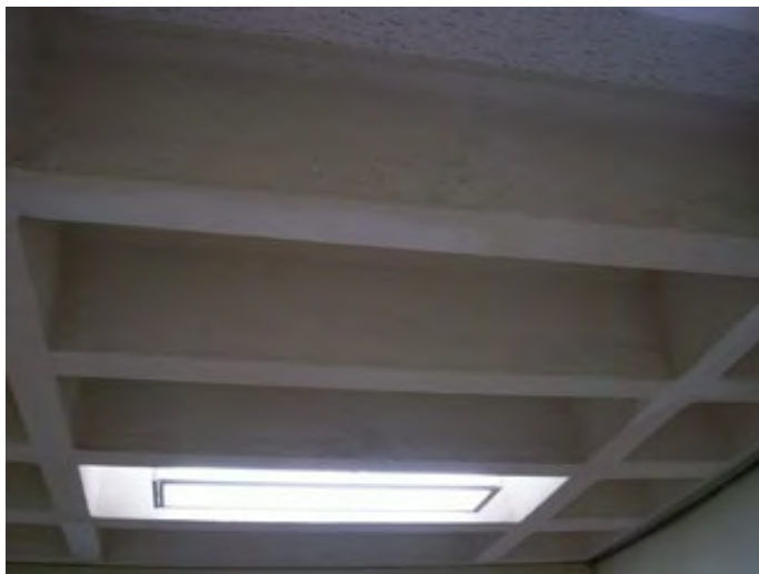
Textured ACM at Cast-in-Place Concrete
