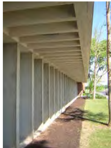
Exposed Concrete Soffit
