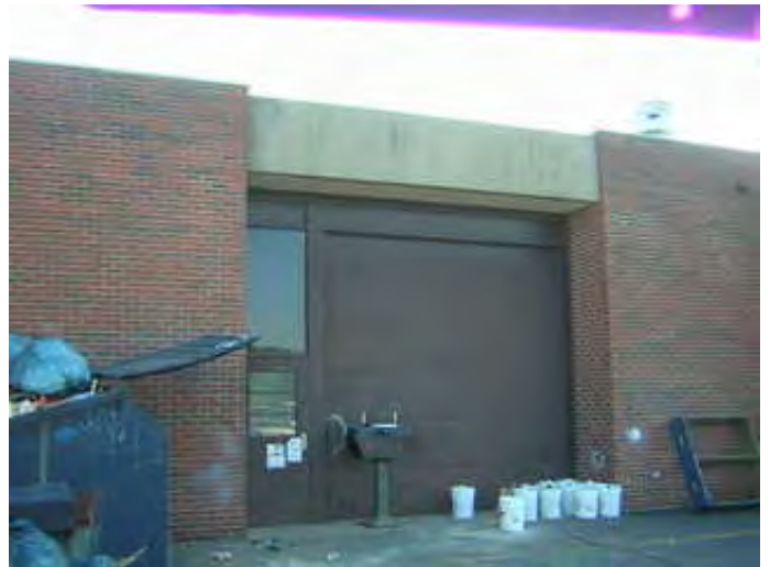
1968 Original Construction HM Door and Steel Overhead Door
