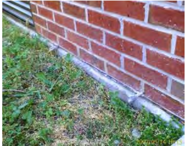
Typical Cast-in-Place Concrete Foundation Wall
